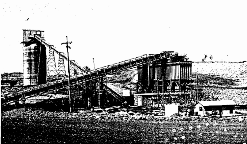
Six Surge Bins and Ring Mills Concrete Silo in Rear
