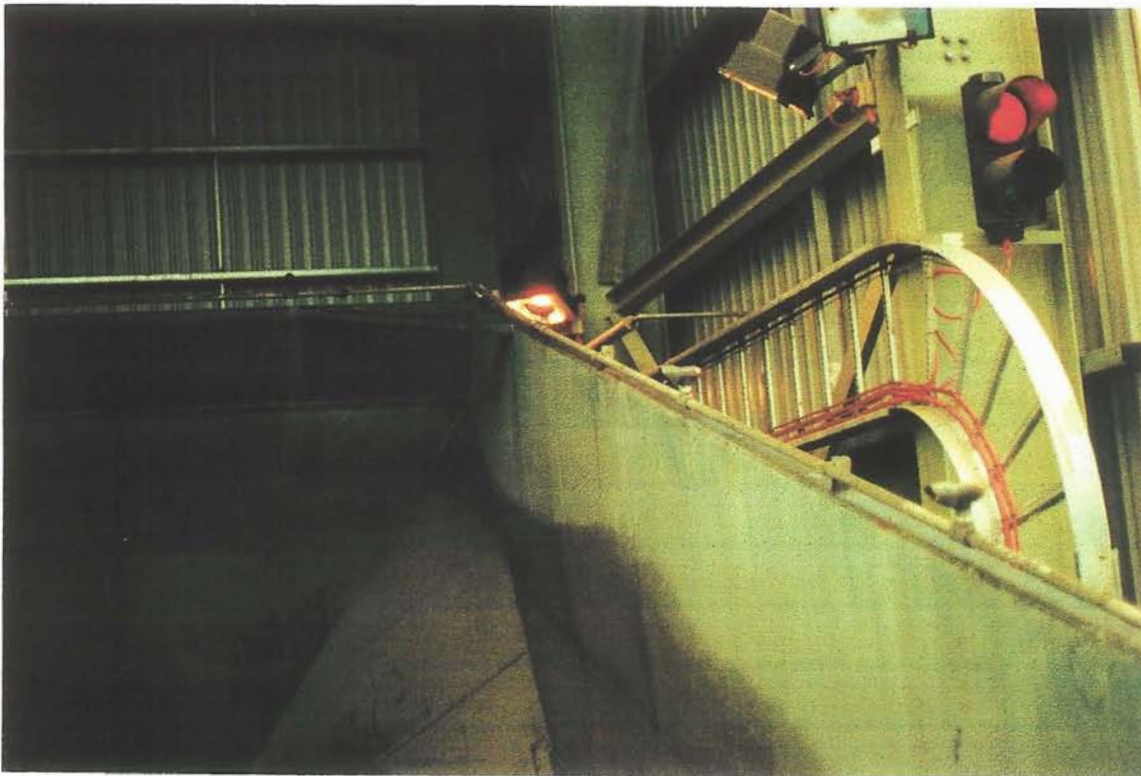
Receiving Hopper (Surface Charger).
